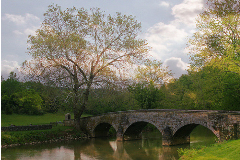
Burnside's Bridge over Antietam Creek
